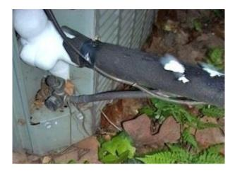
If ice is present here, then it is also possible to have ice on the evaporator coil in the attic. When ice coats the evaporator coil in the attic, air cannot flow past the cold coils—very little air flow will be observed flowing out of the AC registers throughout the house. Follow this procedure to thaw the evaporator coil (this is a short term solution until the system refrigerant can be replenished).
